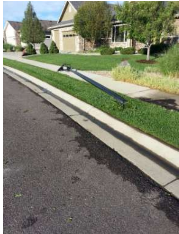
Street lamp blown over during a severe thunderstorm near CoCoRaHS Station CO-BO-271 on August 3, 2013.
