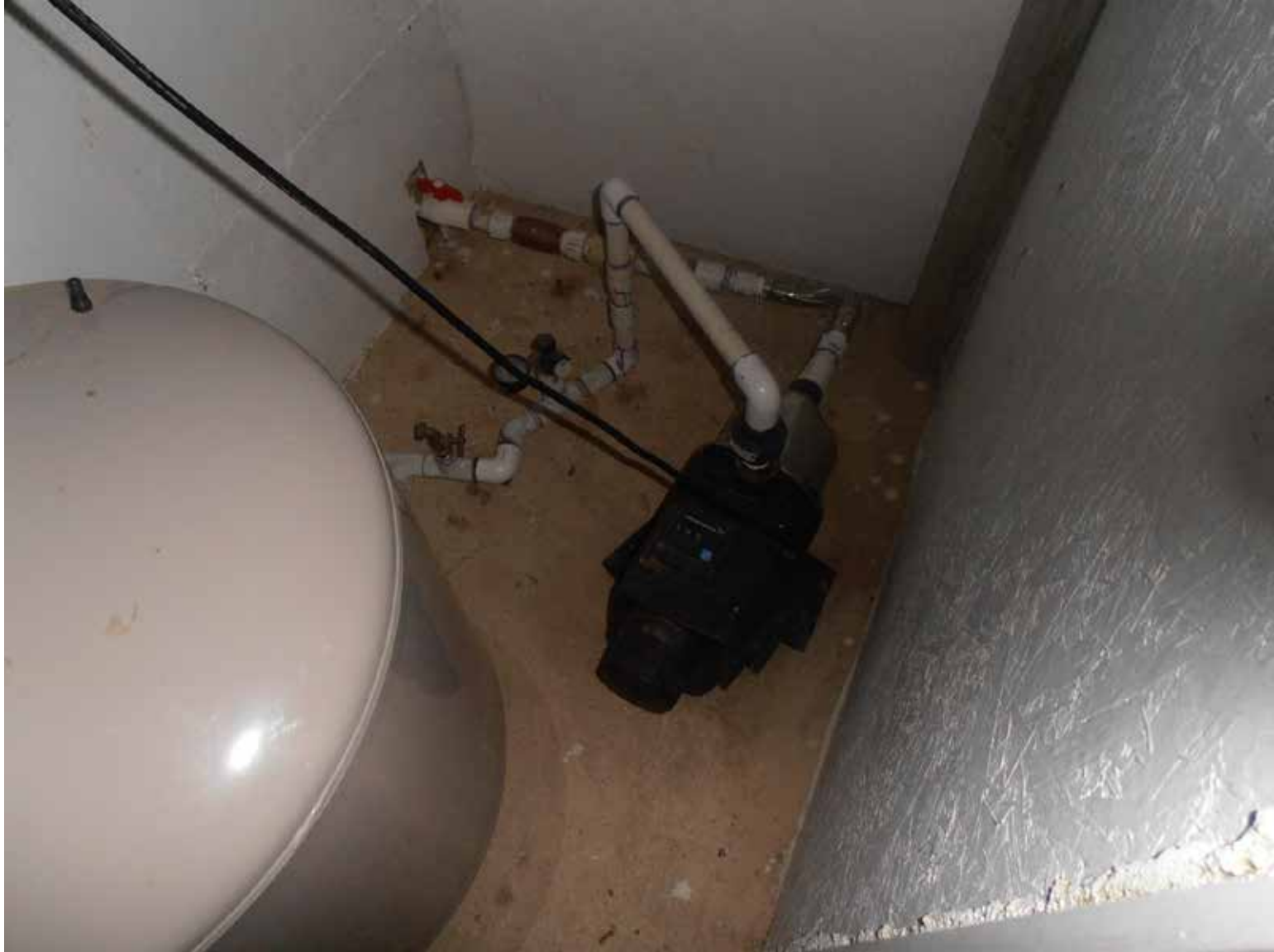
1 horse pump and 40 gallon pressure tank
