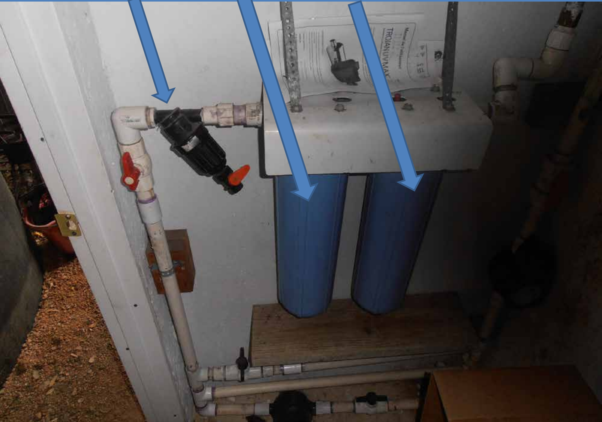
3 filters – 80 micron, 20 micron and 5 micron charcoal filter
