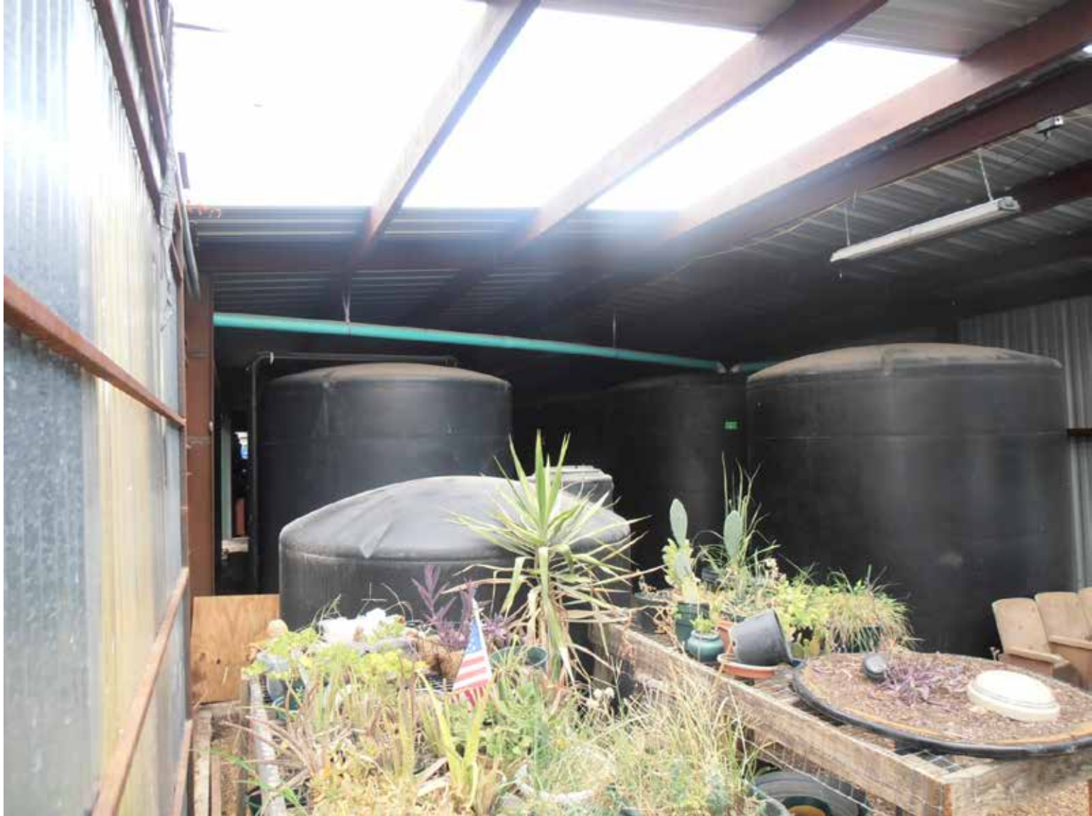
Rain barn – 16,500 gallons storage inside and 9,000 gallons out back. Total 25,500 gallons
