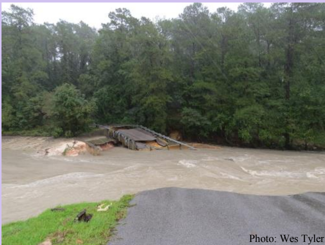
Cary Lake Dam Failure at Skii Lane
