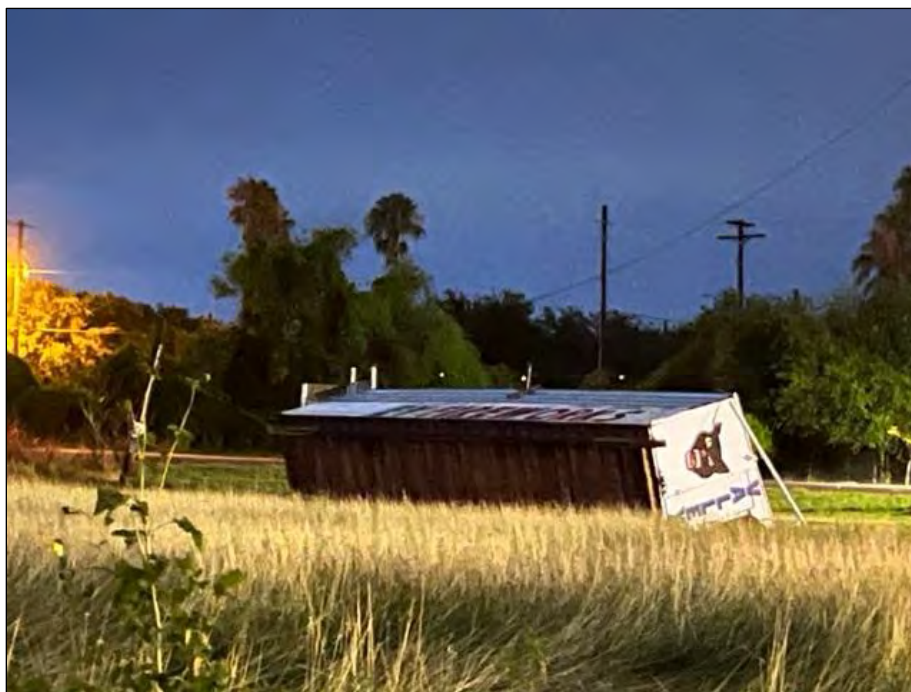
Above photo 1: Flipped fireworks stand in east San Benito, June 4, 2023, from wind gusts estimated at 60 mph. The stand was facing directly into the north wind and not securely anchored.
