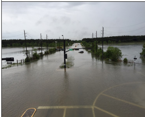
View looking west down FM 529 at SH 99 Grand Parkway.
