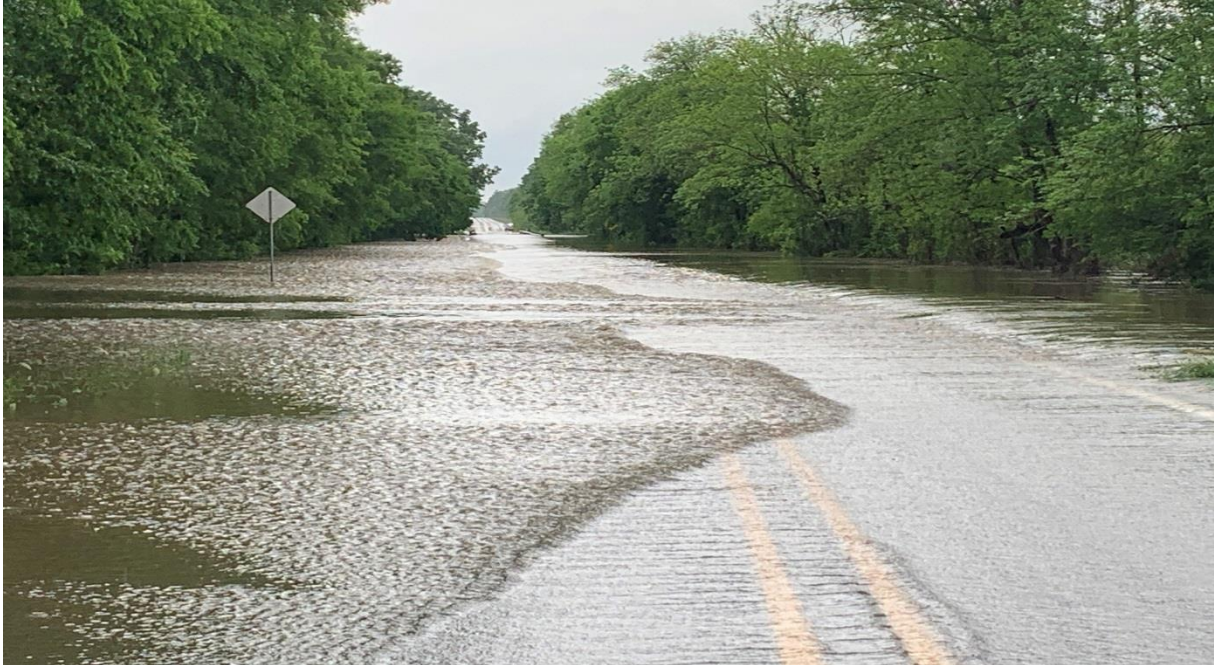
Fig.5: Flooding on FM Road 324 (Angelina County) April 30, 2021 Photo Credit: TXDOT Lufkin
