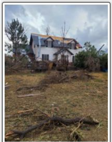
Damage to a home north of Happy (Amarillo OEM)
