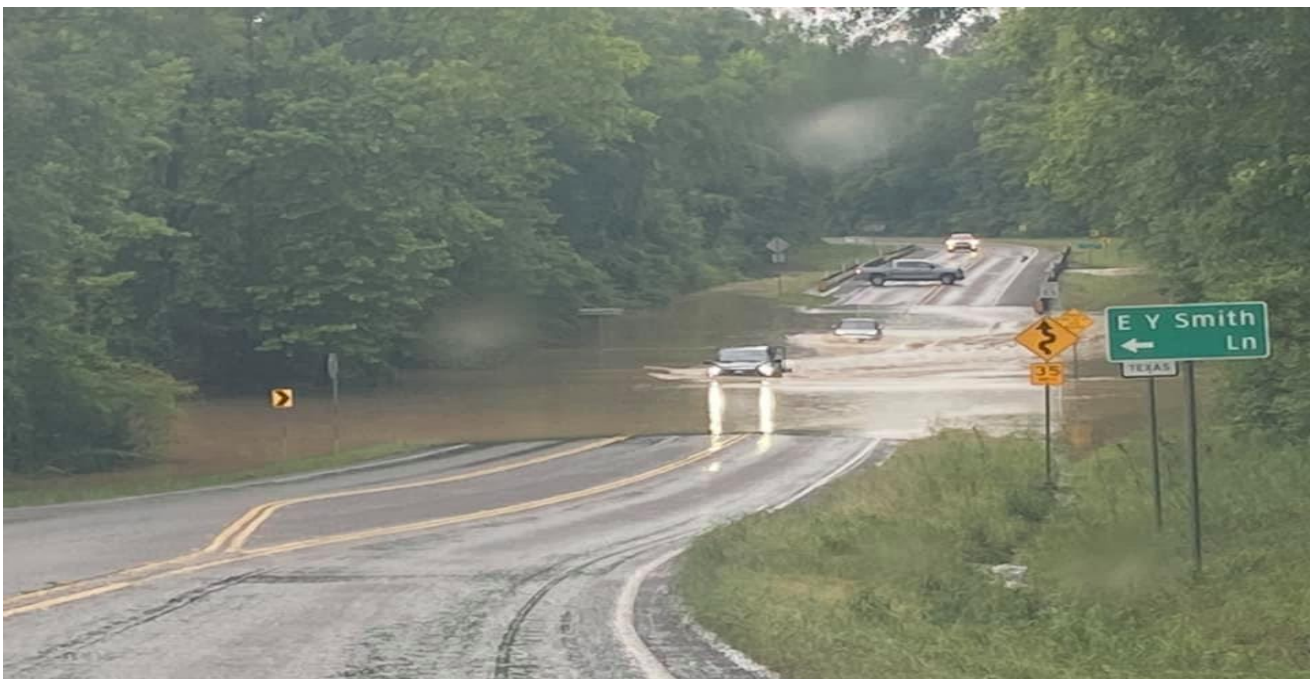
Fig.6: Flooding on State Highway 87 near Fairmount (Sabine County) May 17, 2021 Photo Credit: Sabine County Reporter
