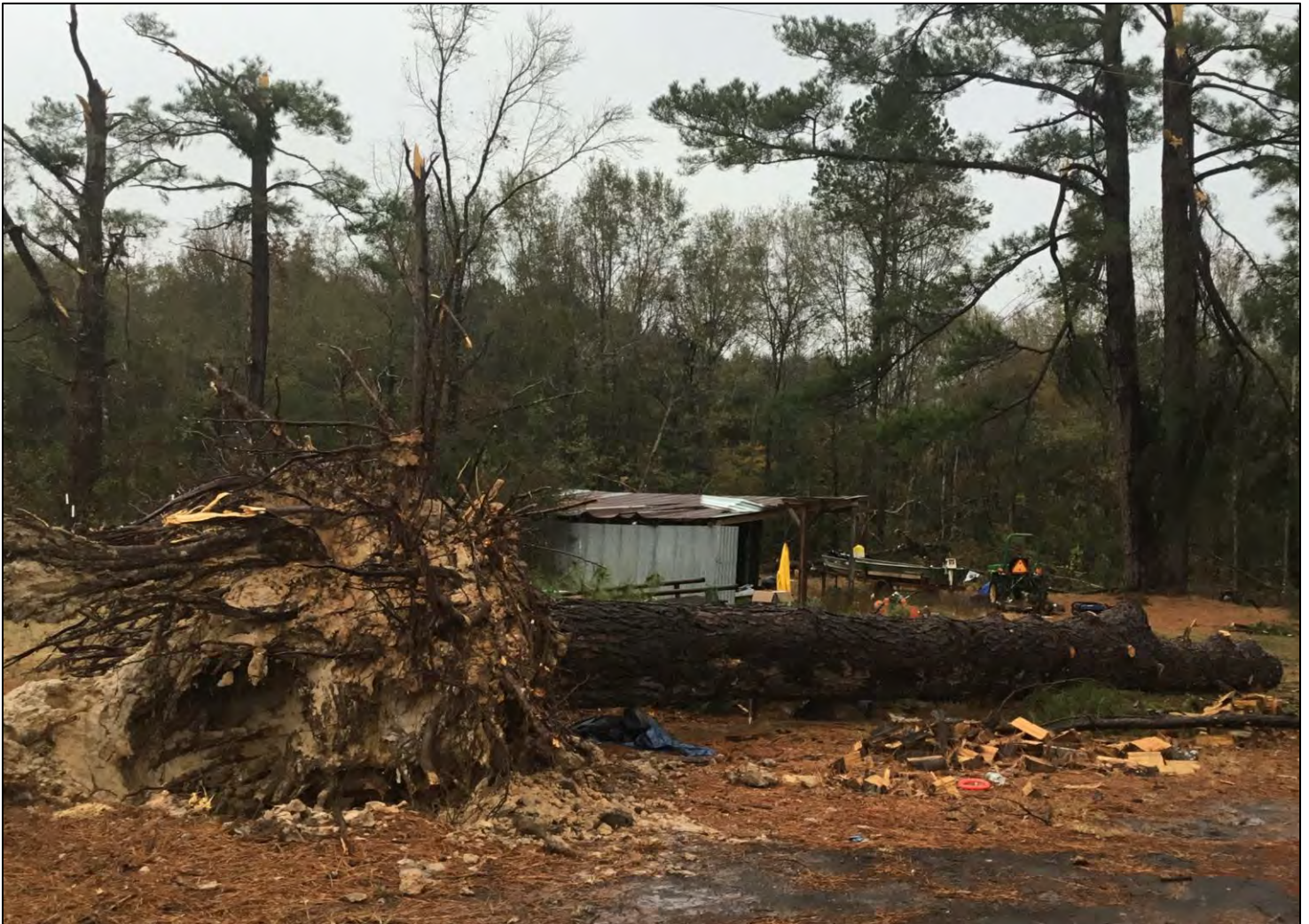
Figure 2: Panola County EF-1 Tornado Damage – November 25, 2020
